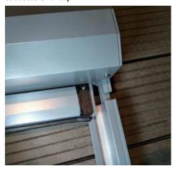
**Step 6**: Putting the zipper track into the guide rail
